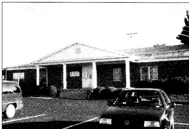
The new National Office in Belleville, IL.
